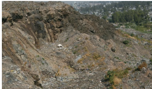
Landfill collapse in Addis Ababa, Ethiopia
