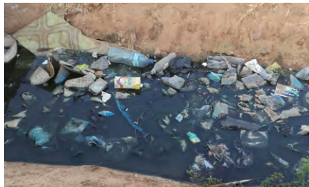
Waste clogging drainage channels
